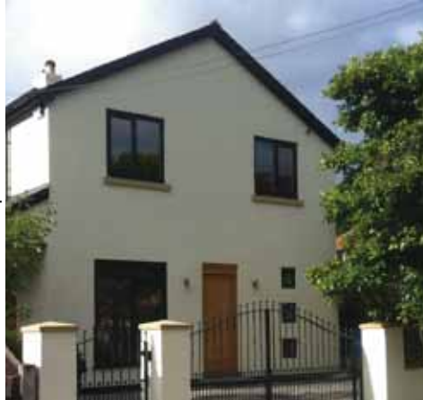
Example of render and dark grey windows in Dalton Grove, Heaton Moor
