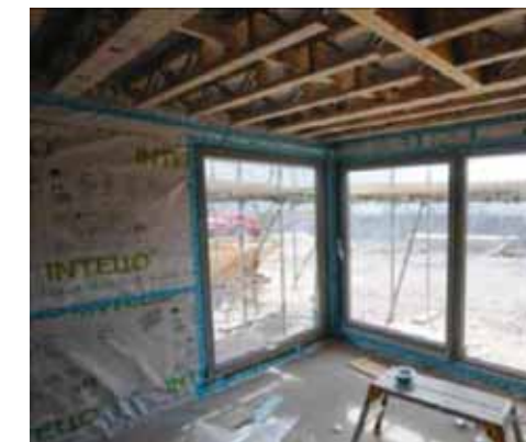
3 Air tight construction using air barriers
